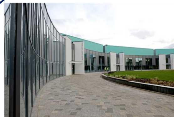
Temporary modular school building
